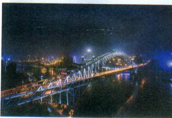
Figure 14.13: The Chaotianmen Bridge over the Yangtze River in Chongqing City, China. The bridge is one of the world's longest through-arch steel bridges and has a span of 552 m.
